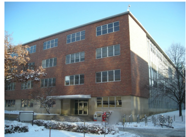
Figure 3: The main building within Robert's major
